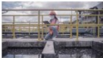
On-site Wastewater Treatment
