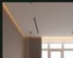
Ceiling POP False Ceiling
