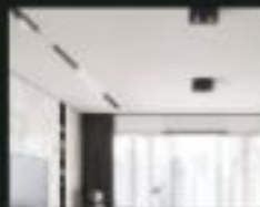
Ceiling POP False Ceiling
