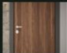
Internal Doors Veneered Polish Door
